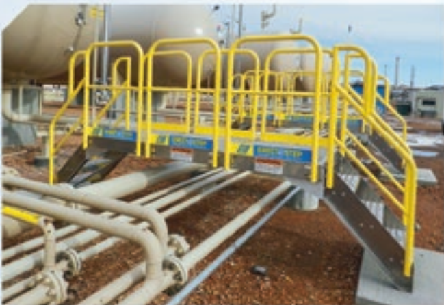
Propane gas lines no longer a safety issue.
