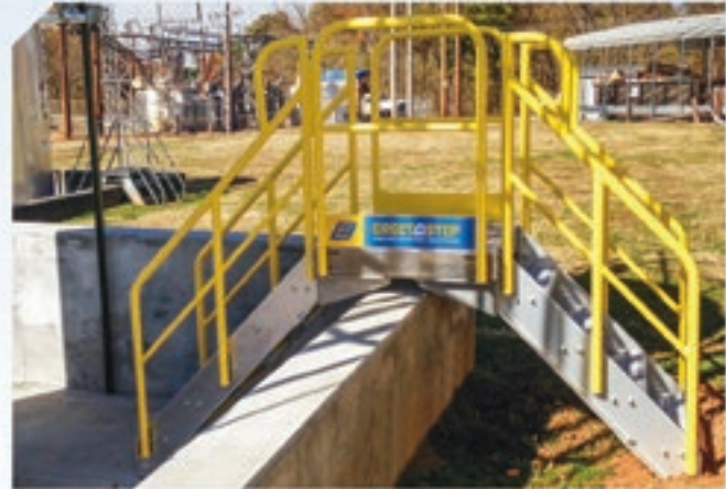
Safely cross containment walls.
