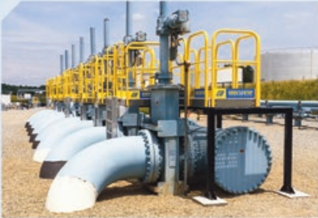
Safe valve access.
