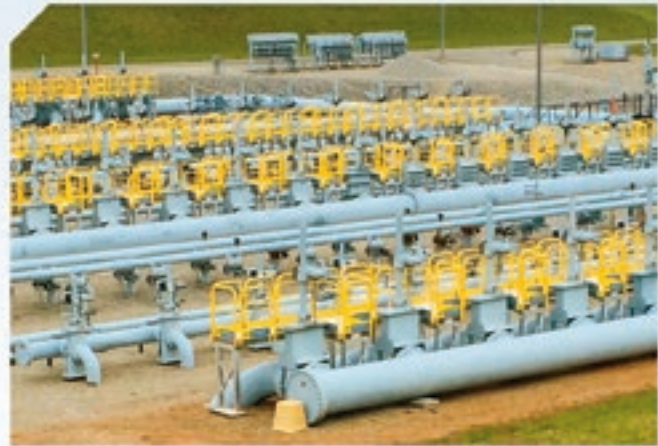
Safely and efficiently access multiple valves.
