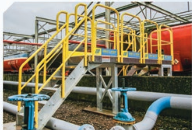
Access over and across multiple obstructions safely.
