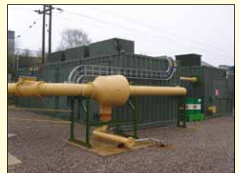
15" KSS Cyclone Separator Natural Gas Application
