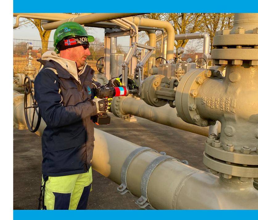
With the EasiDrive portable valve actuator, you easily handle hard-to-operate and time-consuming valves without expensive actuators. For standard valve gearbox sizes, the EasiDrive can be used with an adaptor and reaction kit specifically engineered for seamless integration. It enables fast, efficient operation as a reliable part of the EasiDrive system, making the switch from handwheel to torque tool operation almost instant.
