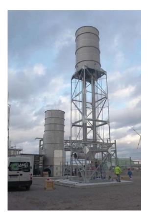
Type: Combustion capacity: Equipment: LTF, biogas emergency flares 50 kW – 60 MW (or more, on request) open combustion (flame visible), integrated ATEX blower, gas train enclosure
